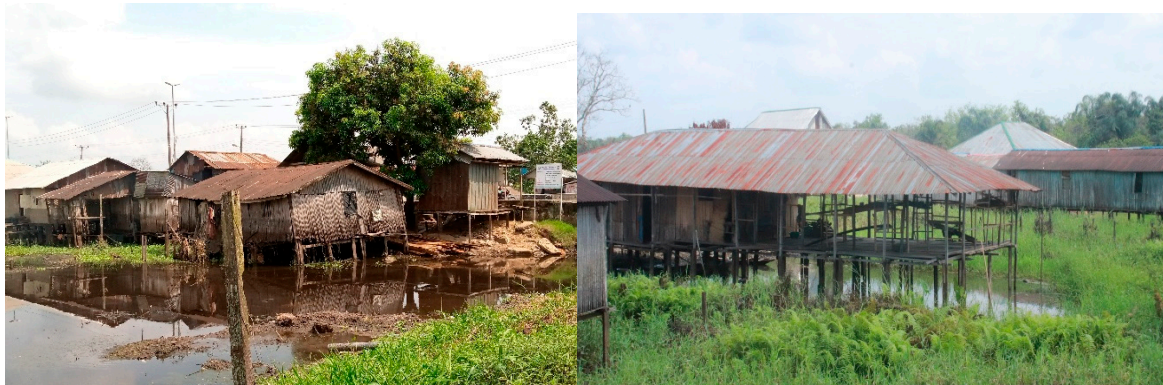
Figure 2. Dwellings on ironwood stilts in Igbokoda, Ondo State, Nigeria.
