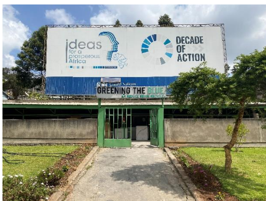
ECA has built a waste recycling center
